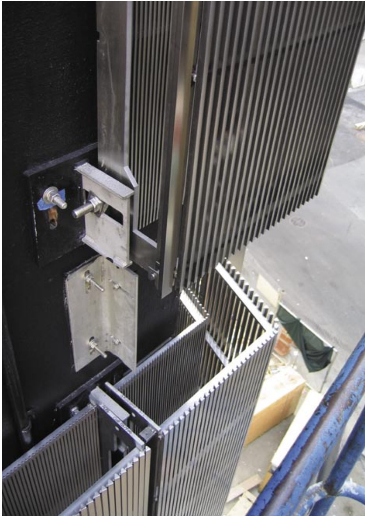
ABOVE Bolted connections anchor the stainless steel screens to the building's concrete exterior.
