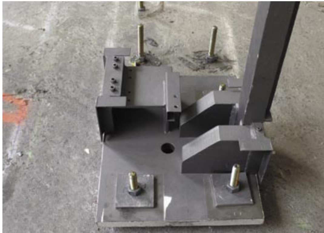
ALL THIS PAGE Highly ductile bridge steel was used for the anchors and supports of the lobby blast wall.
